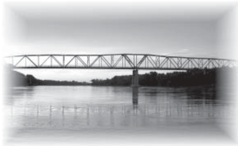
Missouri River Bridge
