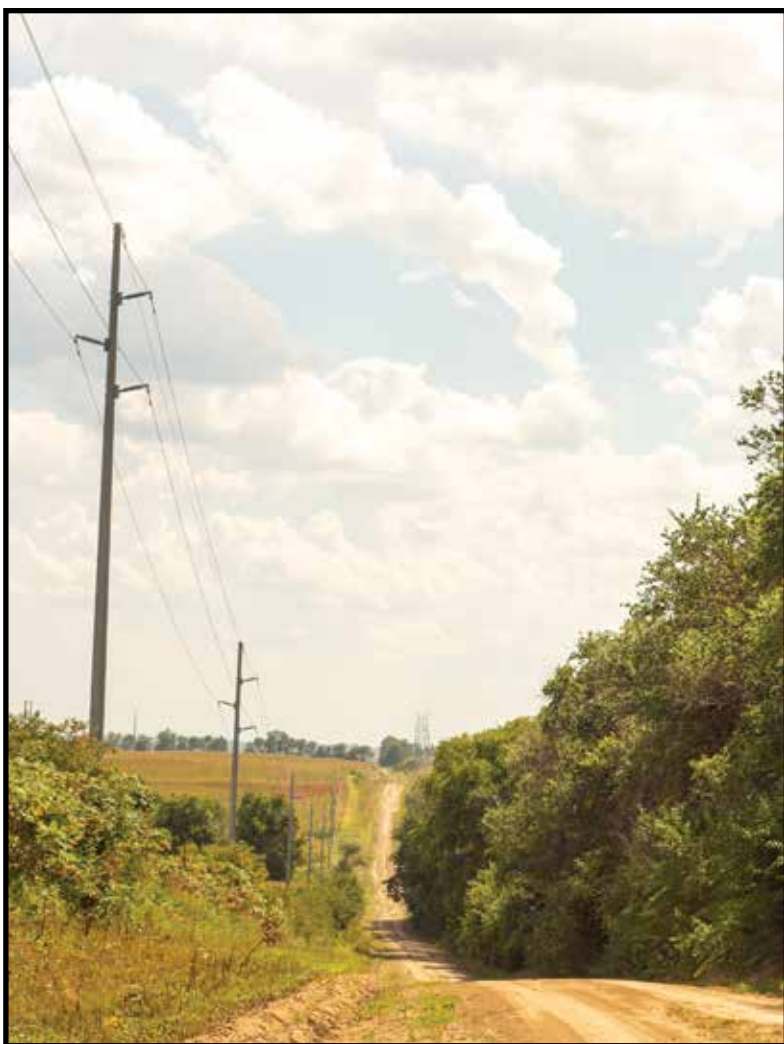
This minimum maintenance road is directly south of Peru.
