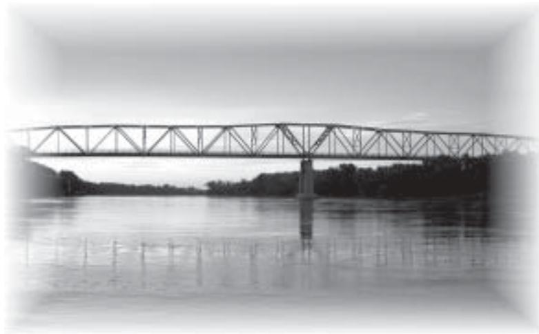
Missouri River Bridge
