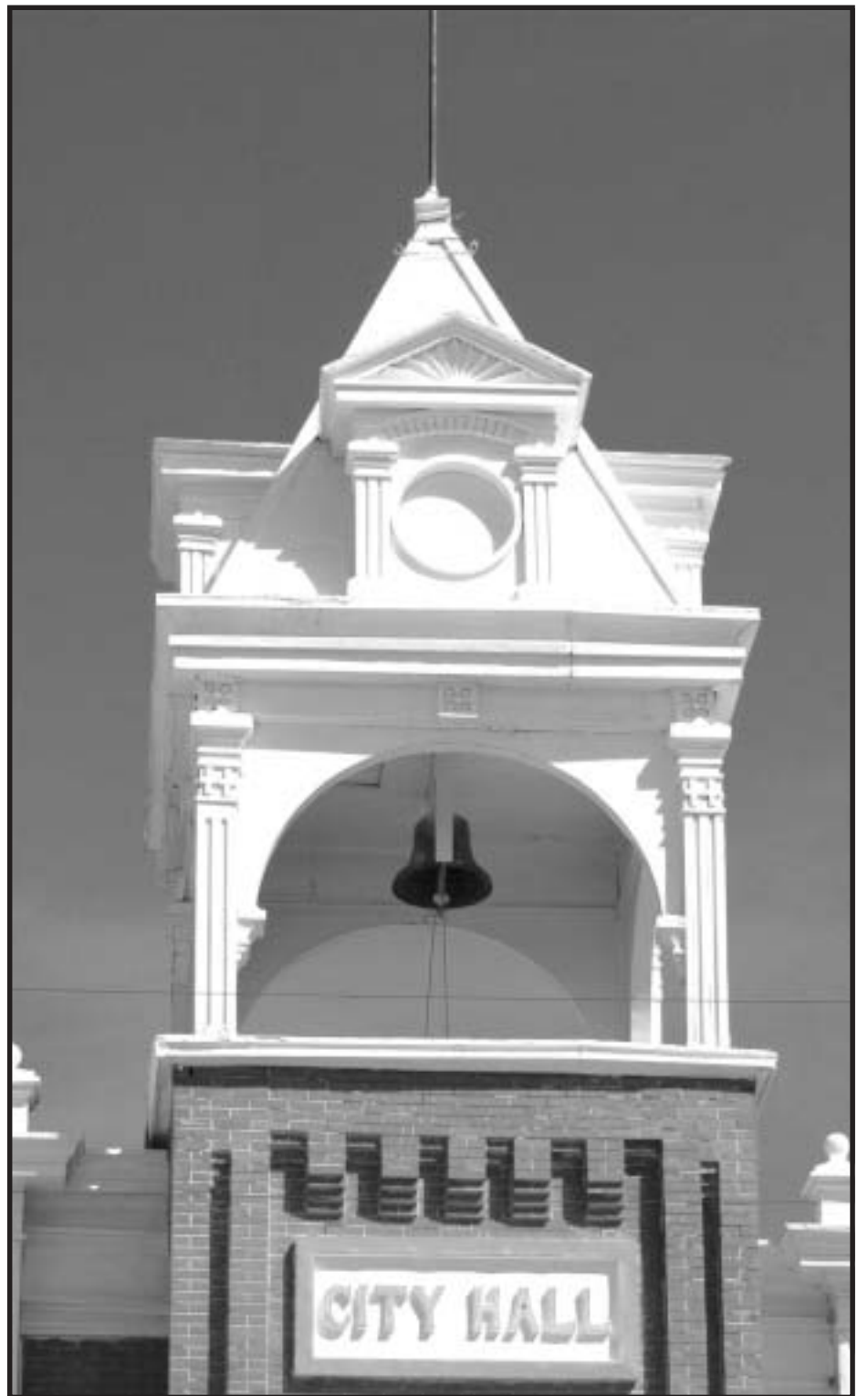
A well preserved city hall.
