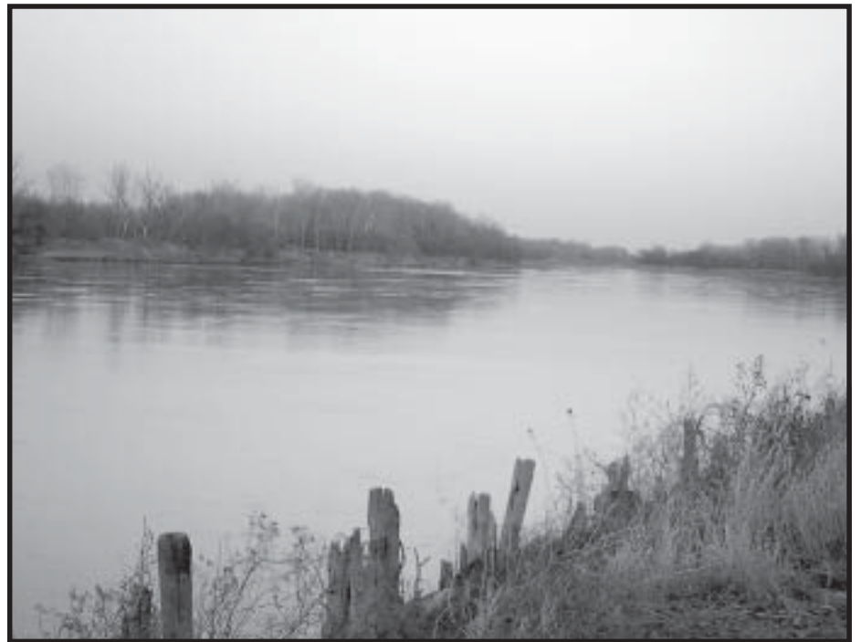
This month's river picture shows the river flow over the top of the rock dikes.
