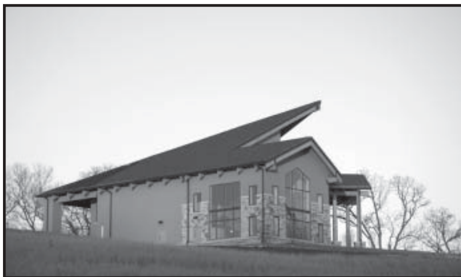
A relatively new structure near what town?
