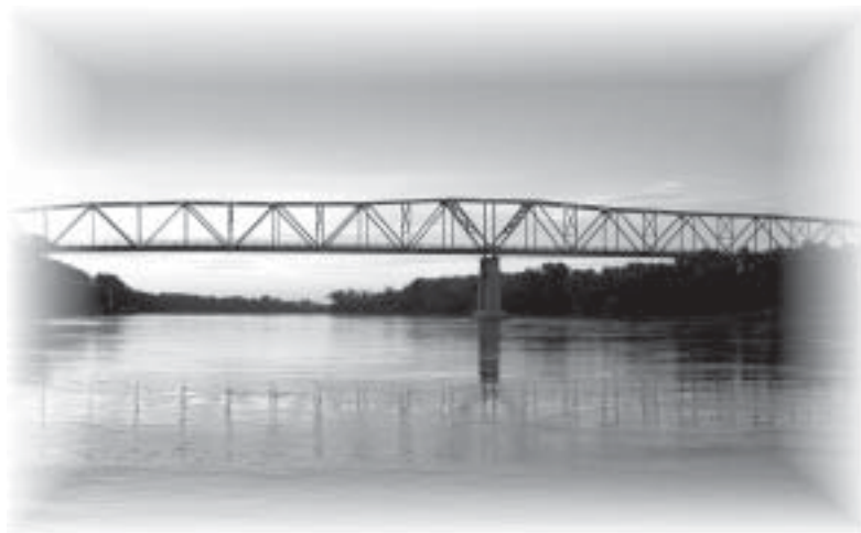
Missouri River Bridge
