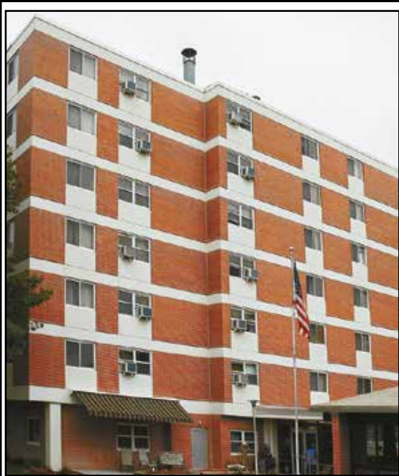
Valley View Apartments (High Rise) • 1017 H Street • Auburn, NE
