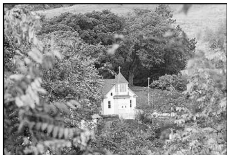
St. Clara's Catholic Church 604 6th Street
