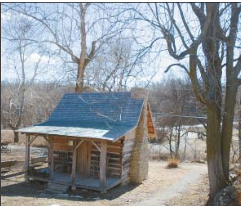
Restored Pioneer Cabin
