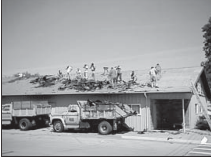
Volunteers roofing the Veterans building.
