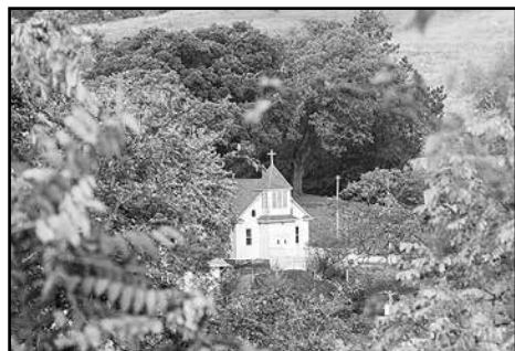
St. Clara's Catholic Church 604 6th Street
