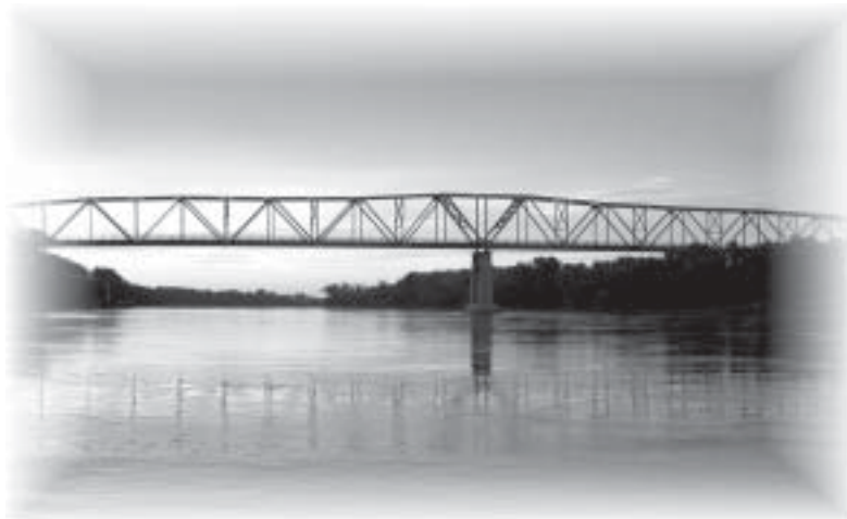
Missouri River Bridge
