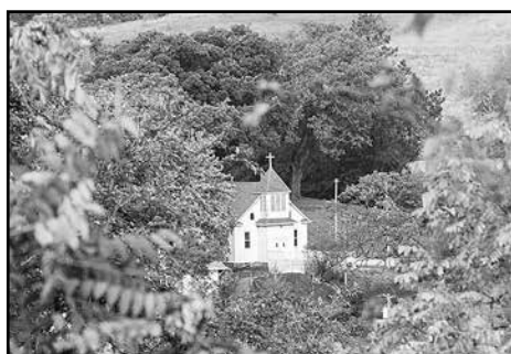
St. Clara’s Catholic Church 604 6th Street
